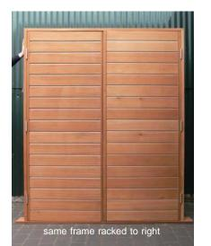
When a frame is pushed slightly out of plumb to the right the doors will be pushed out of alignment with the right door sitting higher
